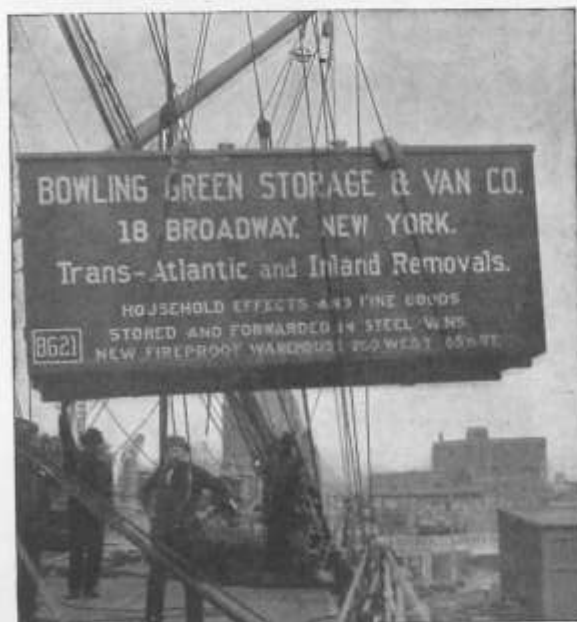
HOISTING LIFT-VAN ON BOARD STEAMSHIP
